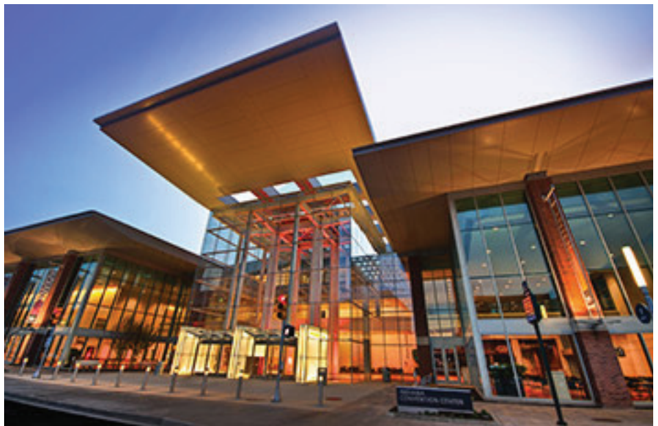
The 2011 expansion added a three-story glass entry pavilion at Capitol Avenue and Georgia Street, and an enclosed walkway between the convention center and Lucas Oil Stadium. (Photo courtesy of Visit Indy)
